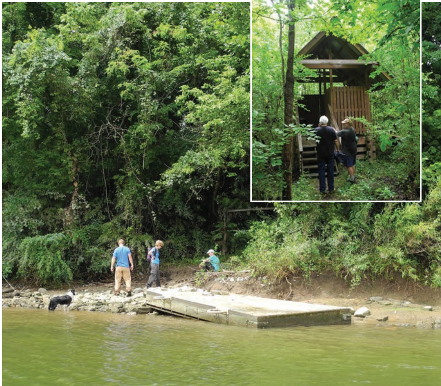
The collapsed dock that is being rebuilt is on the east side of the island. Above inset—a composting toilet.
